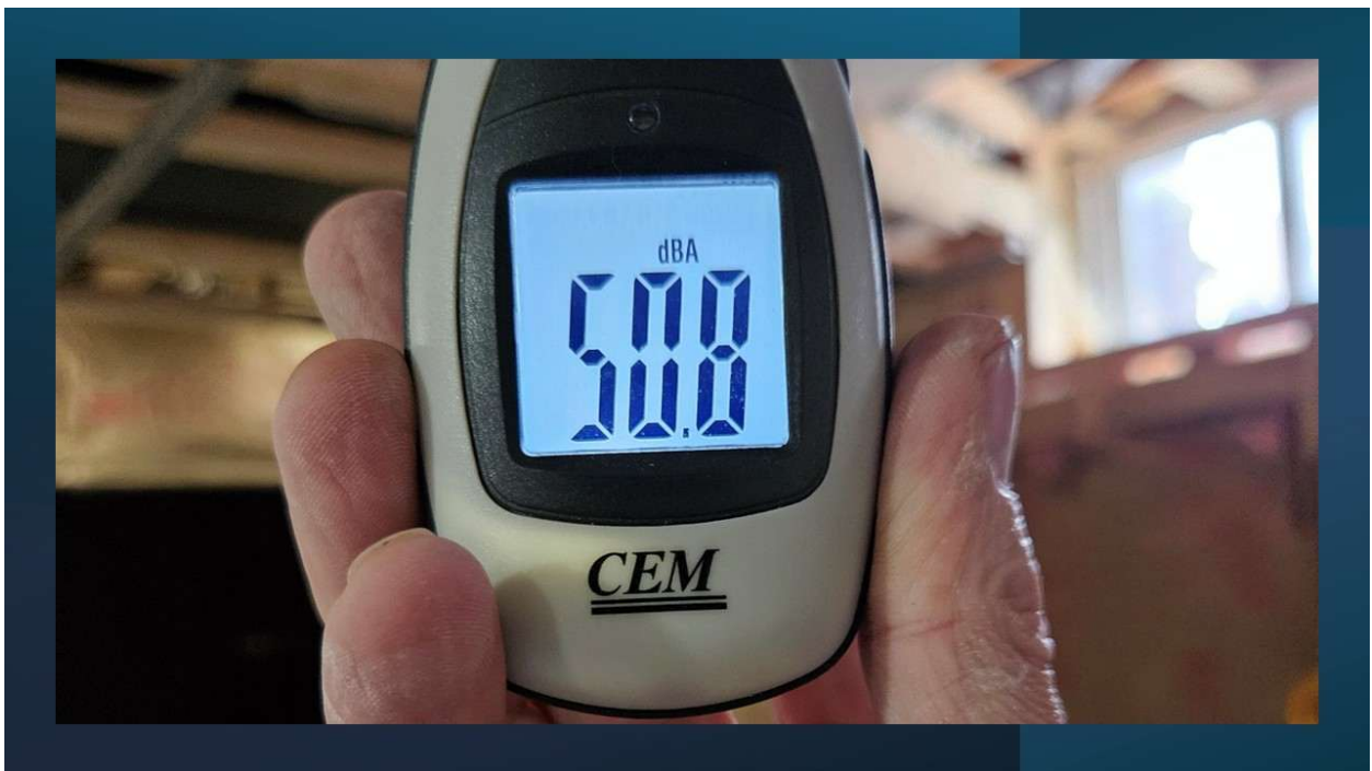
Figure 4: Sound Meter reading 50 db with most of the first layer of drywall in place and 4 inline duct fans above operating
